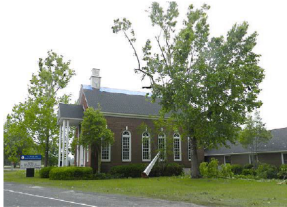
Clarendon County Severe Thunderstorm (church steeple off with downed trees)
